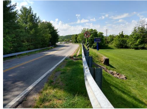
Guard rail between retaining wall and road
