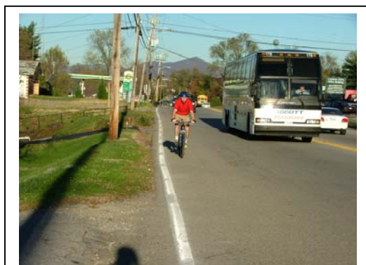
Figure 6.4. Wide travel lane along Colonial Avenue between Broadway and Persinger.
