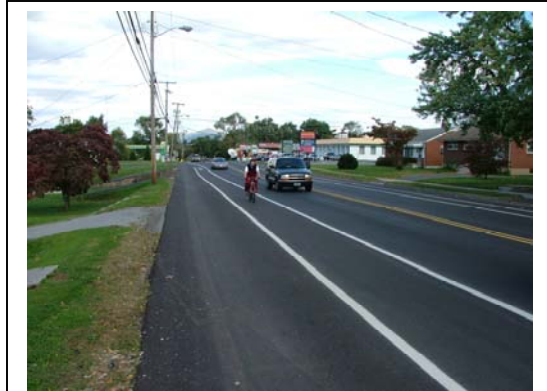
Figure 6.5. Colonial Avenue between Broadway and Persinger after repaving. Note reconfiguration of existing pavement with to accommodated on-street parking and a bike lane.
