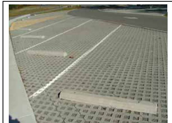
Figure 6. Parking lot in Wasena Park constructed to allow water to infiltrate instead of producing runoff.
