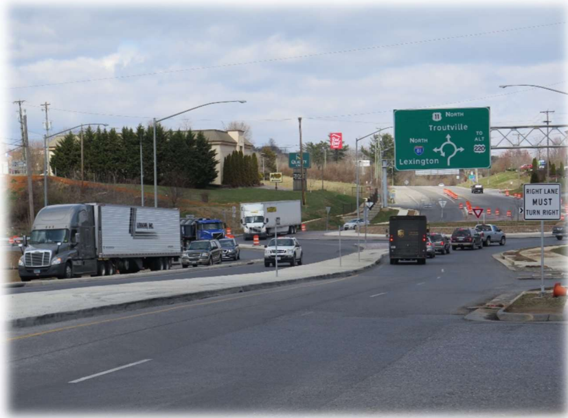
Route 11/I-81 Exit 150/Alt. 220 Roundabout
