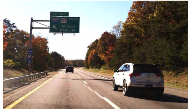
Figure 4- 1 I-81 and I-581 are a key corridors through the Roanoke Valley March 23, 2017
