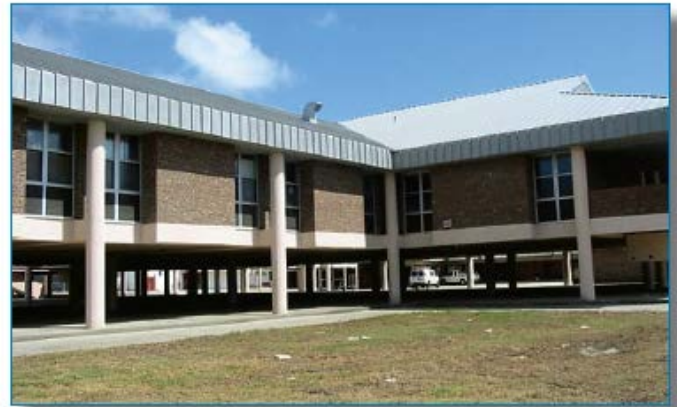
Figure 1: School elevated on columns
