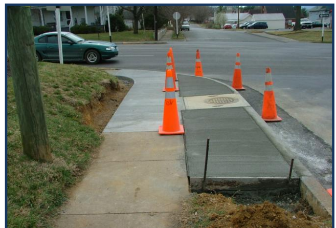
Image 8.5.3 Sidewalk installation at the corner of Virginia Avenue and 3 rd Street.
