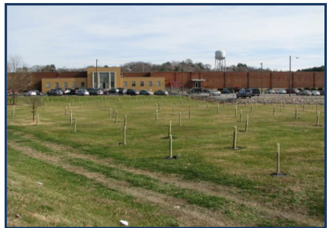
Image 6.4.2 The PFG plant is located on Virginia Avenue near the limits of Roanoke City.
