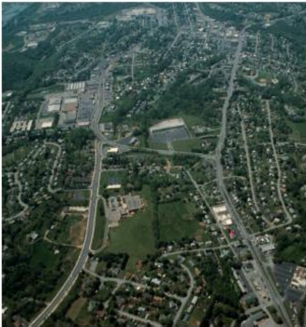
Image 1.0 Aerial view of the Vinton study corridors including: Bypass Road, Washington Avenue and Hardy Road
