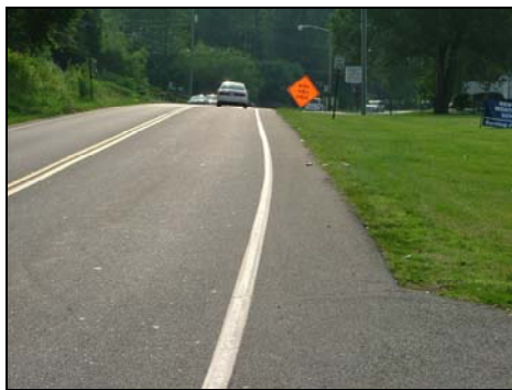
Paved shoulder along Brandon Avenue in the City of Roanoke
