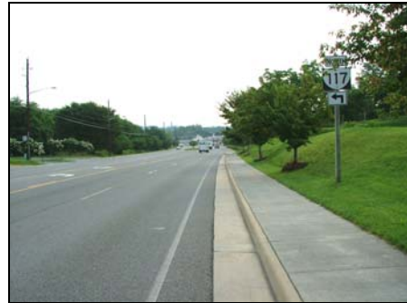
Edge striping creating a 2-foot paved shoulder along Brandon Avenue in the City of Roanoke.
