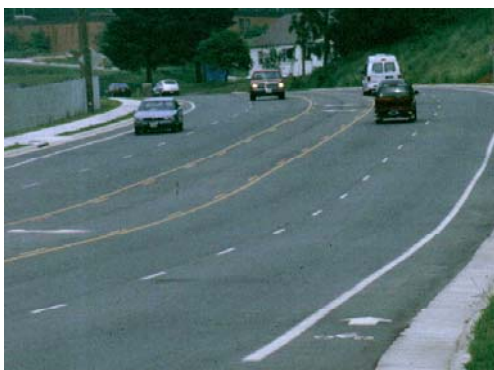
Bike lane with curb and gutter along Hardy Road in Vinton
