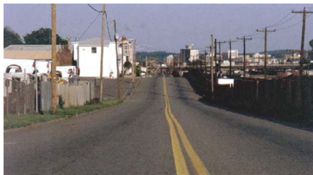
Wide travel lane on Shenandoah Avenue in the City of Roanoke
