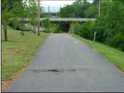
Roanoke River Greenway, paved surface
