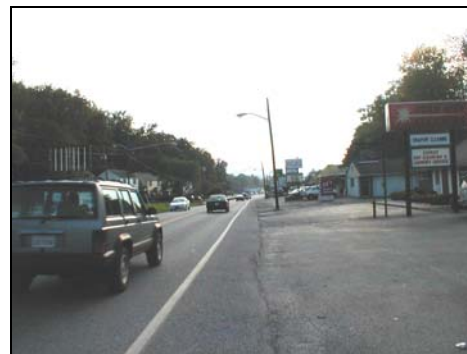
Paved shoulder on Brambleton Avenue
