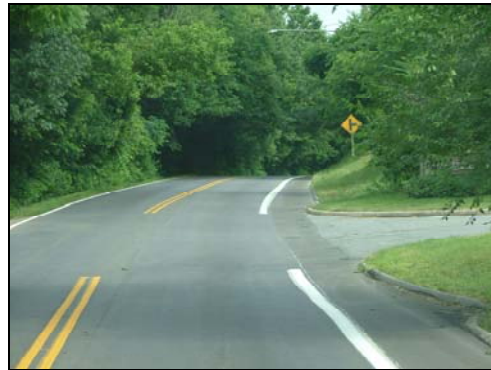
Paved shoulder along the Salem Bike Route
