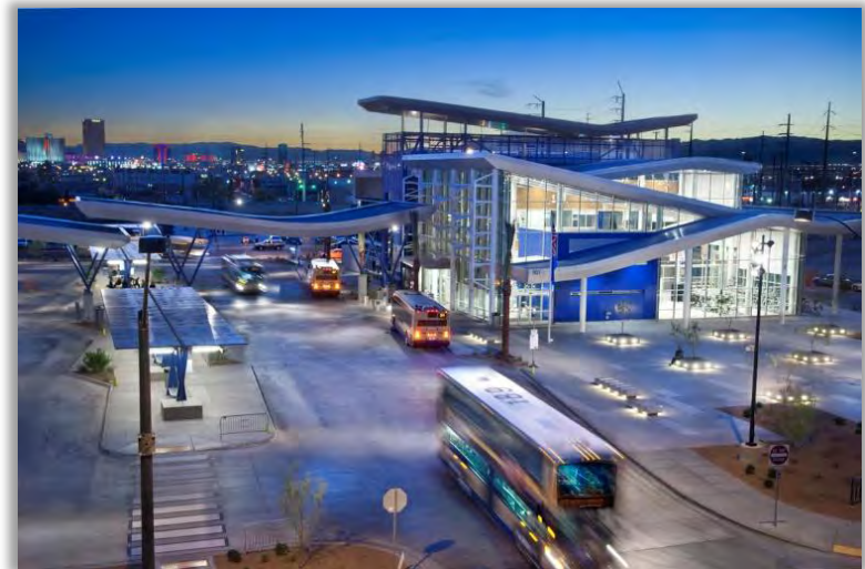
Figure 7.1-3 | Example of Large-Scale Transit Transfer Facility in Las Vegas
