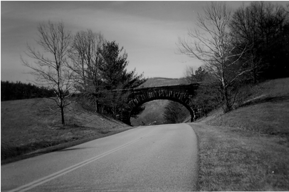
Blue Ridge Parkway in Roanoke County
