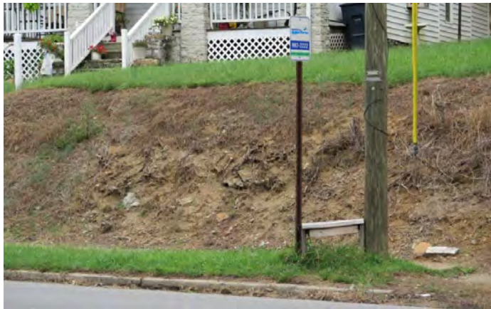
Figure 7.1-2 | Makeshift pedestrian facilities at bus stops
