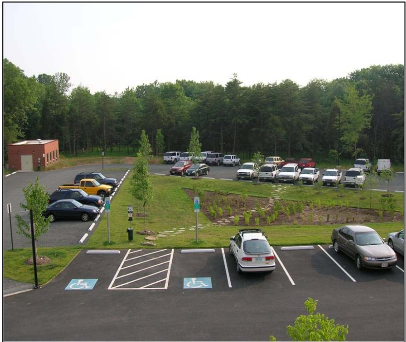
Bioretention Area, Wetland Studies and Solutions, Inc., Virginia (Photograph courtesy of VADEQ)
