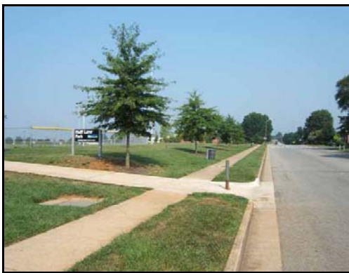
Former design of sidewalk entrance to Huff Lane Park.
