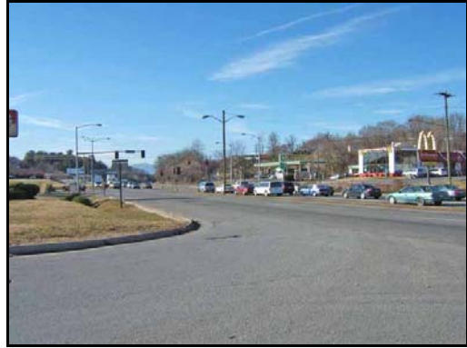
Route 460 and King Street intersection.
