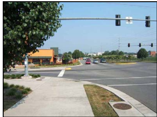
Lack of crosswalk at intersection of the Ring Road and Valley View Boulevard.
