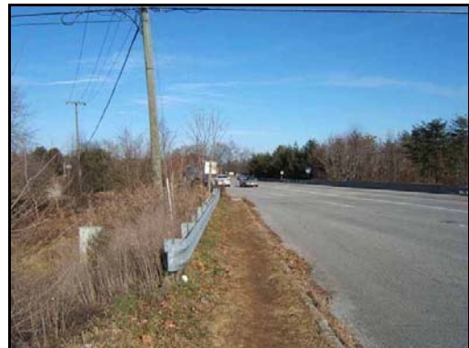
Existing path along Ogden Road.
