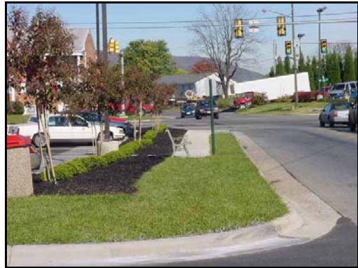
End of sidewalk on Vinyard Road.
