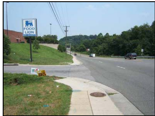
Existing sidewalk along Shenandoah Avenue lacking crosswalks.
