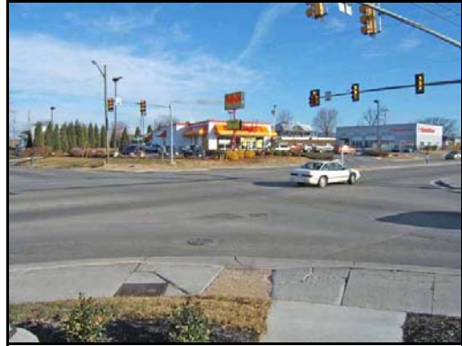
Lack of crosswalks at intersection of Vinyard Road and Virginia Avenue.
