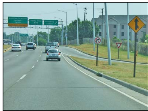
Path along south side of Hershberger Road near Interstate 581 ramp.
