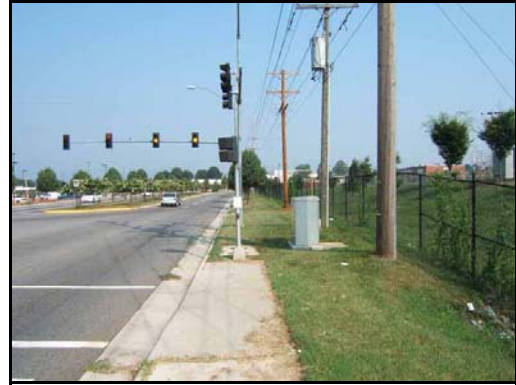
Crosswalk at Valley View Boulevard and Huff Lane Park entrance. Pedestrian signal button and crosswalk in place.
