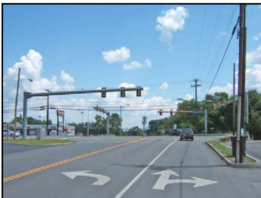
Intersection of Carriage Lane, Grandin Road and Route 419.
