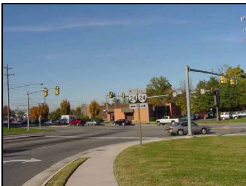
Route 24 Bypass and Hardy Road. Signalized, sidewalks without crosswalks.
