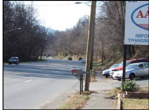
Sidewalk terminates at Transmissions America.
