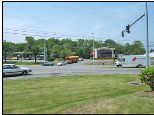
View of King Street and Route 460 intersection.
