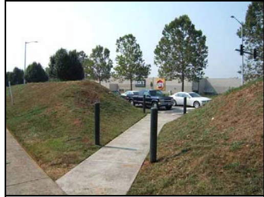
Sidewalk from Huff Lane to Valley View Boulevard NW.
