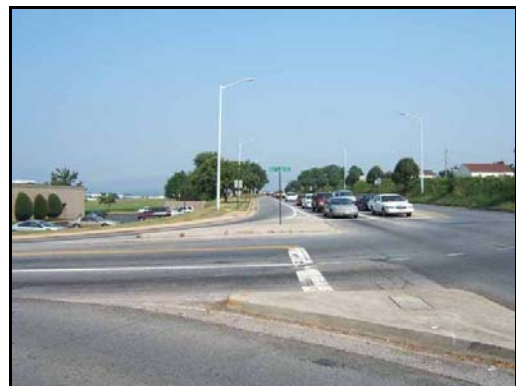
Lack of crosswalk at Valley View Boulevard.
