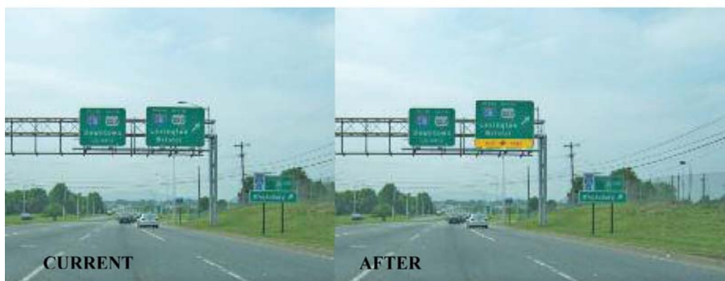
Figure 38-Hershberger Road exit only lane to I-581 north could benefit by better marking on an overhead sign or on the pavement
