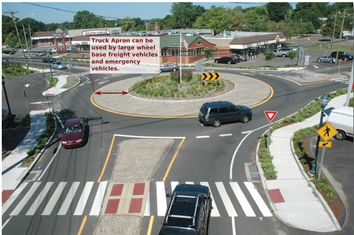
Properly Designed Roundabout with truck/emergency vehicle apron. Roundabout location West Haven, CT designed by William Britnell, original image (without illustration and callout box) provided by VDOT central office, Richmond VA.
