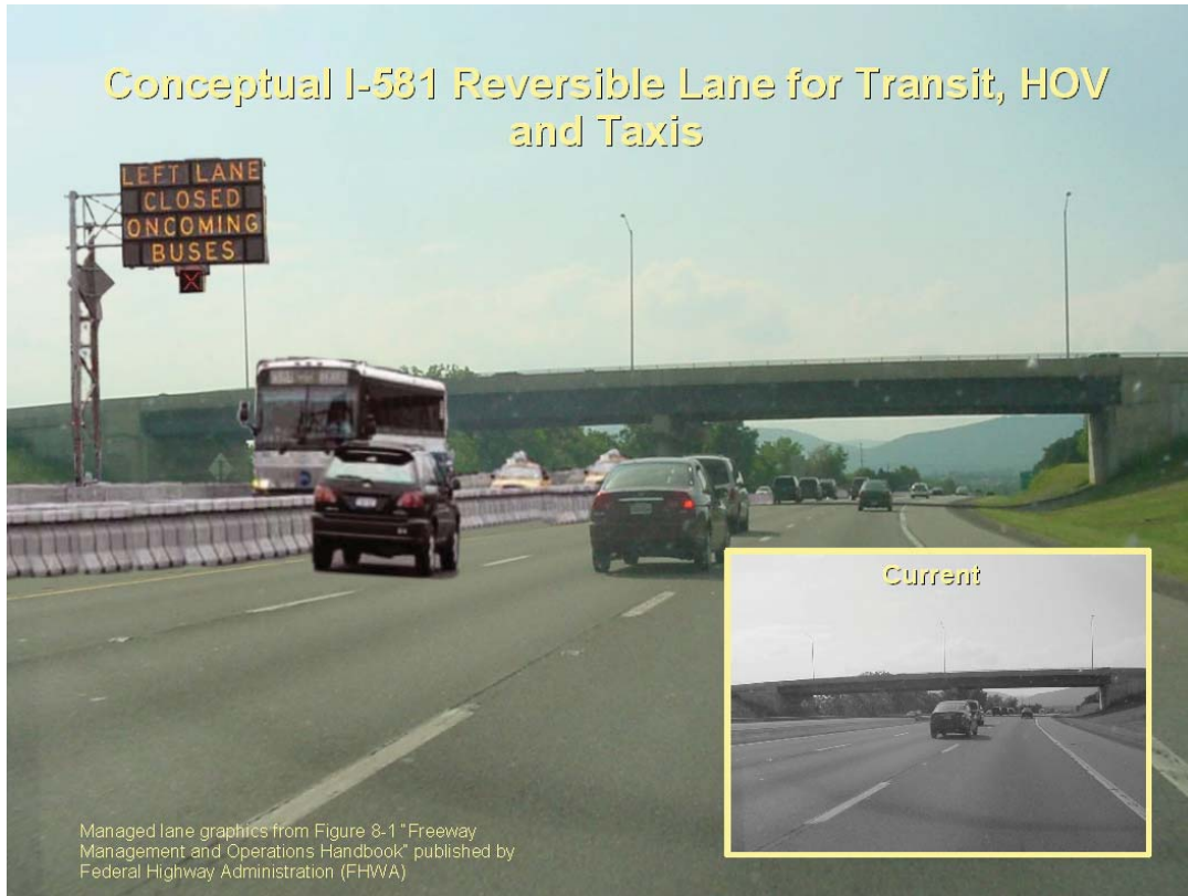
Photo-Simulation of Conceptual Interstate Reversible Lane system on Interstate 581 - Actual Conditions Depicted in Box Labeled "Current"
