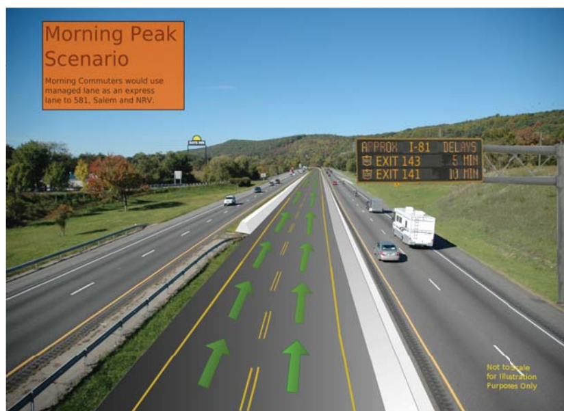
Photo-Simulation of managed lanes in current I-81 median configured for morning peak commute into Roanoke Metropolitan Area. Managed lanes could be coupled with a Variable Message Sign (right).
