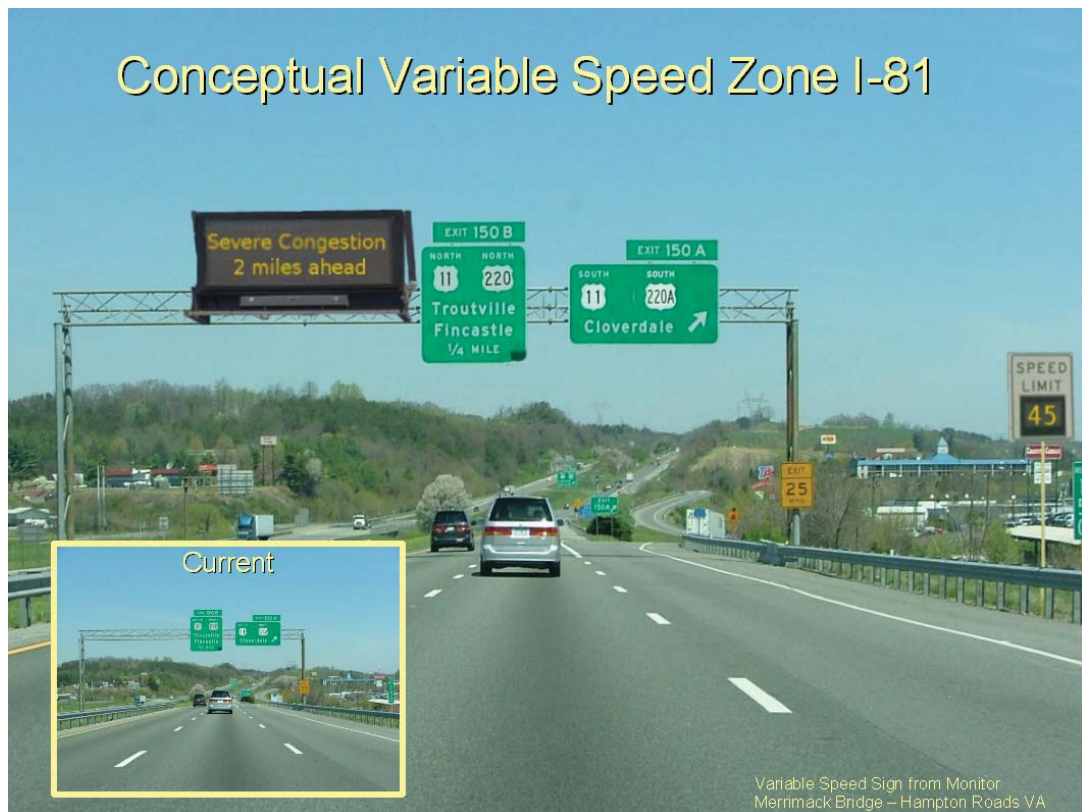
Photo-Simulation of Conceptual Interstate Variable Speed Limit Zone on Interstate 81 - Actual Conditions Depicted in Box Labeled "Current"
