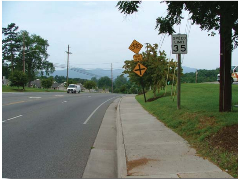
The wide travel lanes, right edge stripe, and Share the Road signage on Brandon Avenue in the City of Roanoke provide separation between cyclists and motorists.
