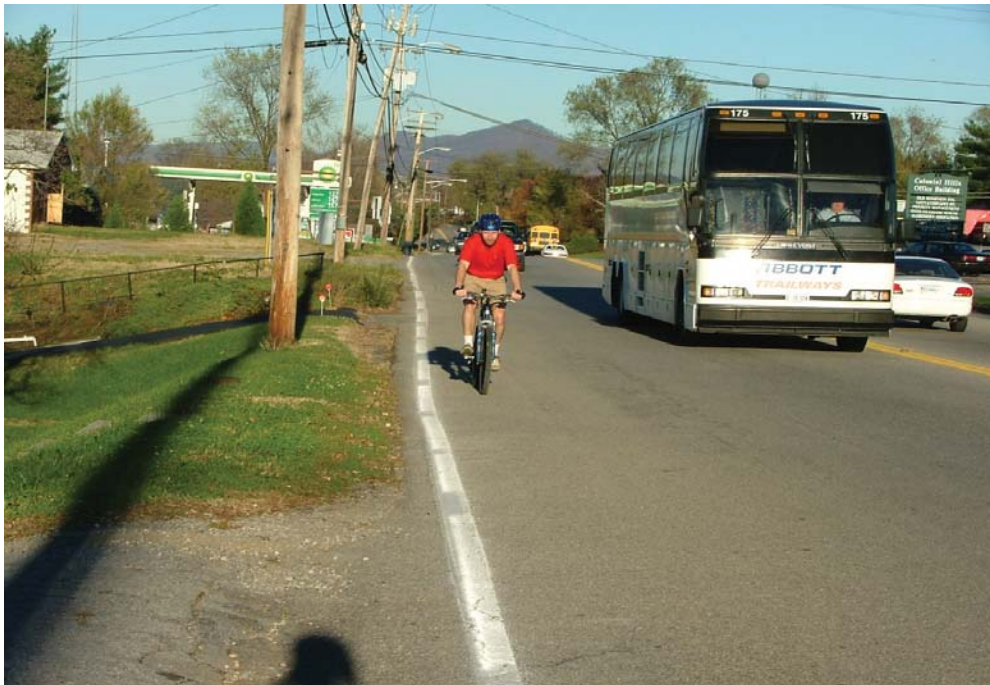
Colonial Avenue BEFORE. A high traffic volume arterial in the City of Roanoke. BCI level of service was D (moderately low) and E (low).
