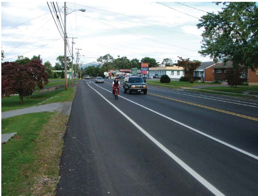
Colonial Avenue AFTER. Re-configured existing roadway width. Narrowed travel lanes, provided bike lanes, and kept on-street parking. BCI level of service rose to C (moderately high).
