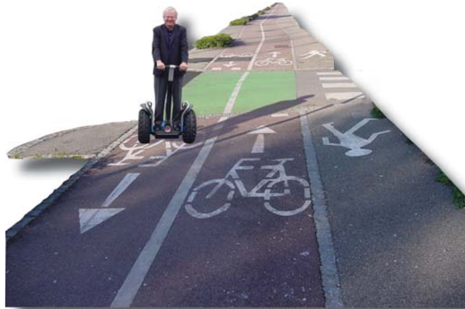
Each lane is 4 feet wide for a total of 12 feet - equivalent to a vehicle lane.
