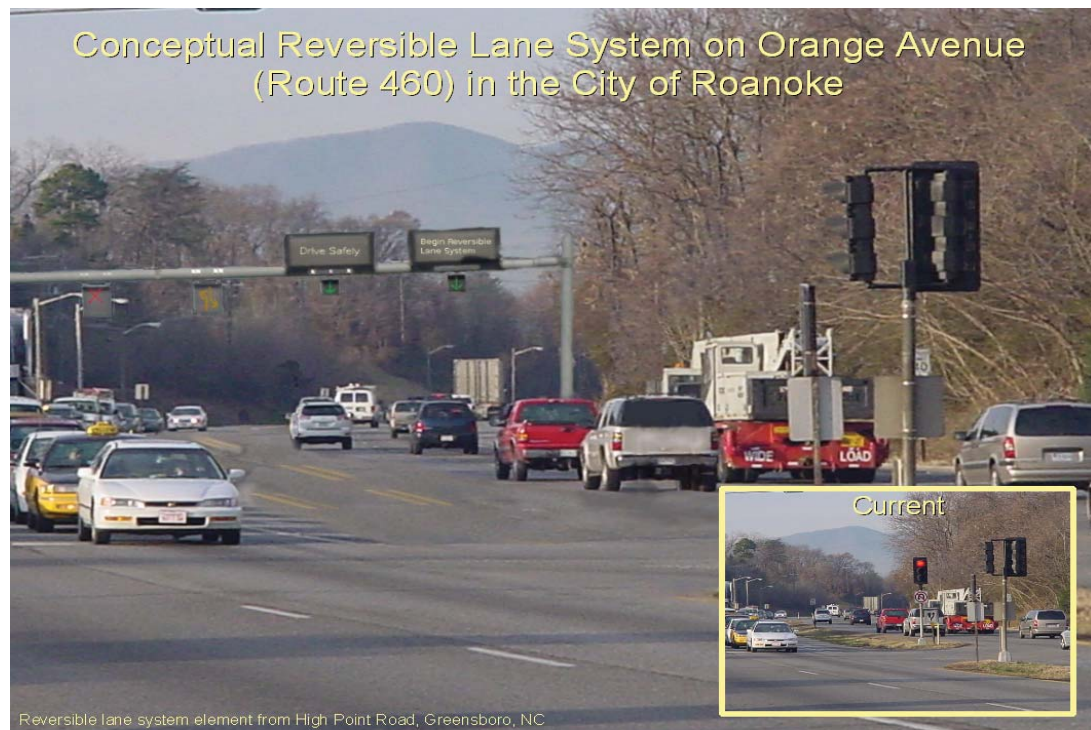
Reversible lane system element from High Point Road, Greensboro, NC Photo-Simulation of Conceptual Reversible Lane system on US 460 (Orange Avenue) - Actual Conditions Depicted in Box Labeled "Current"
