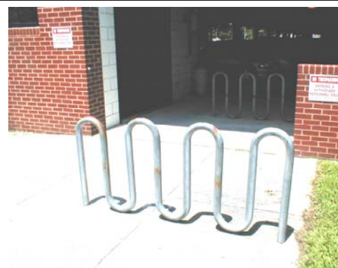
Bike racks at the Williamson Road parking garage. Note that two racks are available – one located outside of the garage and one located inside of the garage protected from the elements.
