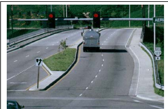
Wide outside lane along Peters Creek Extension in the City of Roanoke.
