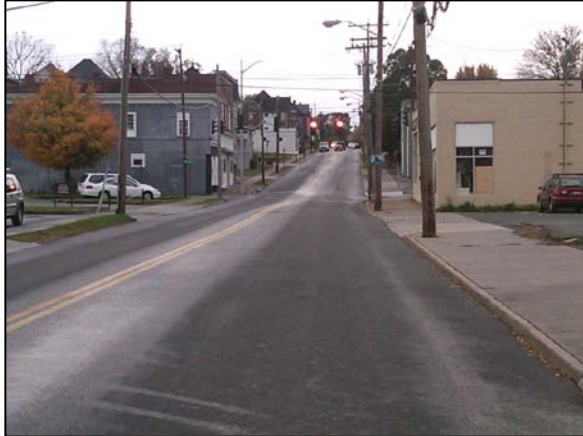
Wide travel lane (road diet) on 5 th Street in the City of Roanoke installed as part of the 2011 annual paving program
