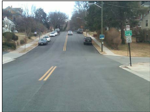
Center line shifted and downhill travel lane narrowed to install wide travel lane in uphill direction on Walnut Avenue/Mill Mountain Greenway (City of Roanoke)
