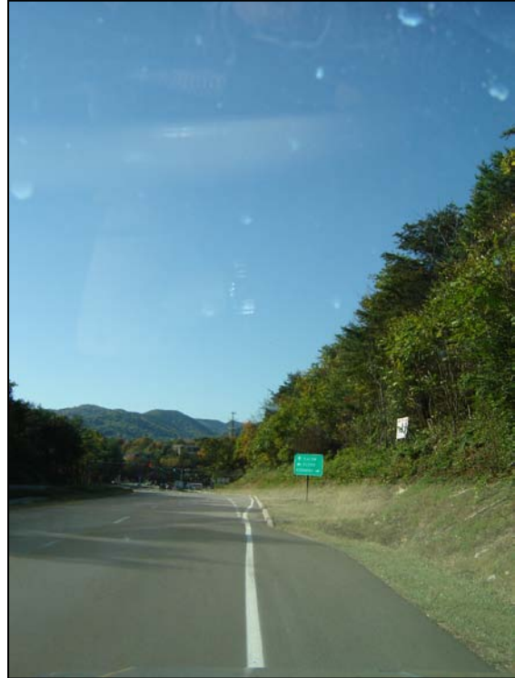
Inconsistent paved shoulder along Electric Road/419 in Roanoke County
