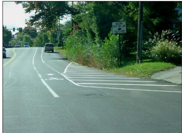
Bicycle lane on Colonial Avenue (City of Roanoke) installed as part of the 2008 annual paving program
