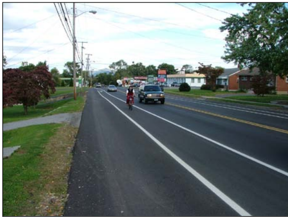
Bicycle lane on Colonial Avenue (City of Roanoke) installed as part of the 2008 annual paving program
