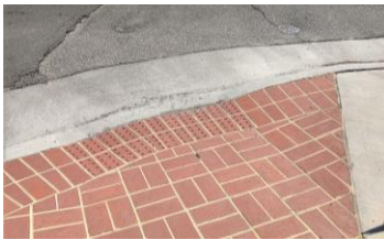
Tactile surface on curb ramp
