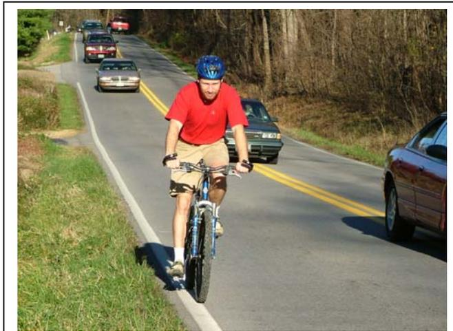
Colonial Avenue between WCL and 419/Electric Road. Note insufficient lane width to accommodate cyclist and auto traffic, and steep gradient.
