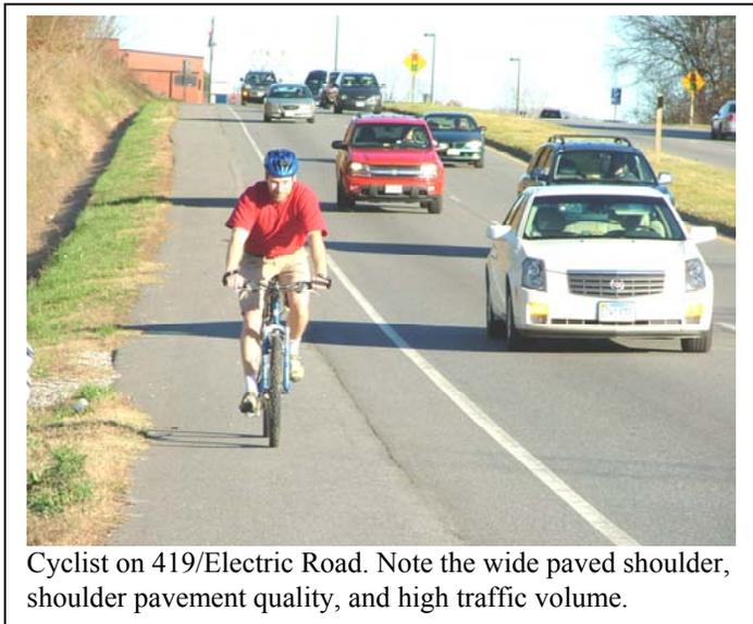
Cyclist on 419/Electric Road. Note the wide paved shoulder, shoulder pavement quality, and high traffic volume.
