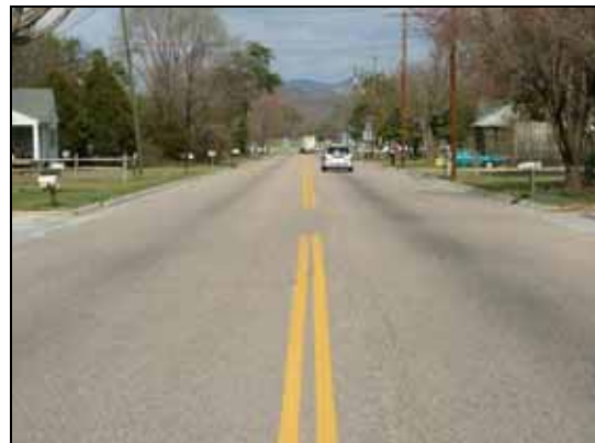
Figure 5.5: Wide travel lane on US 60 Business in Clifton Dale Park, Alleghany
