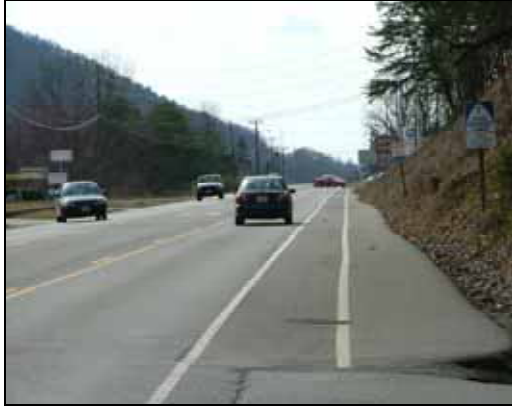
Figure 7.5: Paved shoulder on US 60 Business in Clifton Forge.
