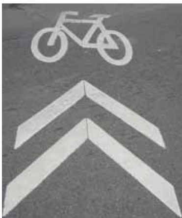
Figure 5.11: “Sharrow” shared lane pavement marking.
