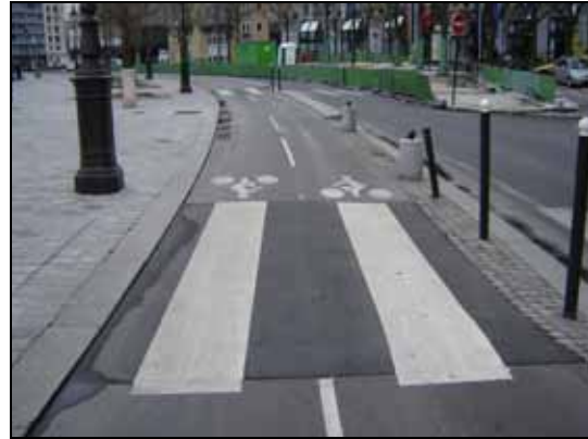
Figure 5.14: Separated bike lane and pedestrian crossing
