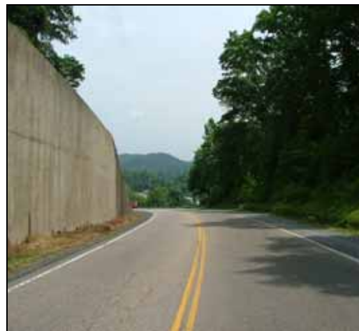
Figure 7.4: Paved shoulder on US 60 in Allegheny County near Clifton Forge.
