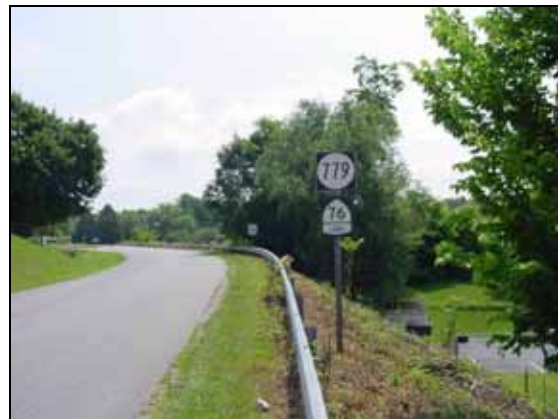
Figure 5.1: Route 779 - Shared roadway typical of the many rural roads.
