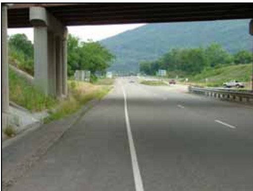
Figure 7.7: Paved shoulder on Route 60 / 220 near Dabney Lancaster Community College.
