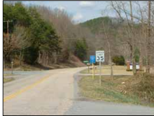
Figure 7.2: Route 629 (Douthat Road) in Allegheny County.
