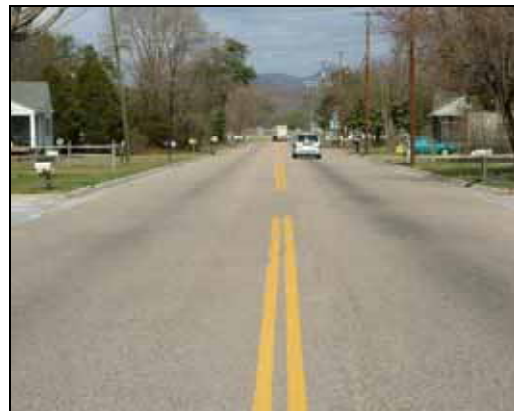
Figure 7.3: Wide travel lanes on US 60 Business in Clifton Dale Park.
