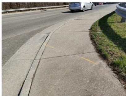
Curb ramps on the segment lack level landing area, tactile surface, and point into the street.
