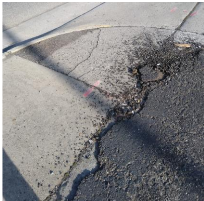
Uneven transition from asphalt
