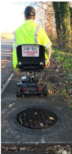
Overcome Yours! Garrett Brumfield navigates his mobility scooter over the storm drain which is elevated >1 inch above the pavement
