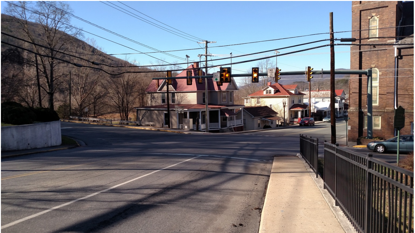
4-way crosswalk markings at Main St & A St lack visibility for approaching vehicles
