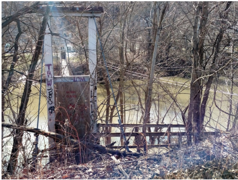
CSX swing bridge over the Jackson River
