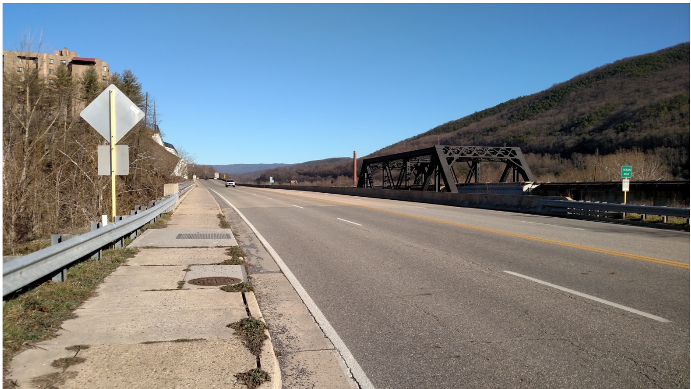
Ridgeway St at Jackson River bridge facing east – bike lanes are recommended in place of the outer travel lanes
