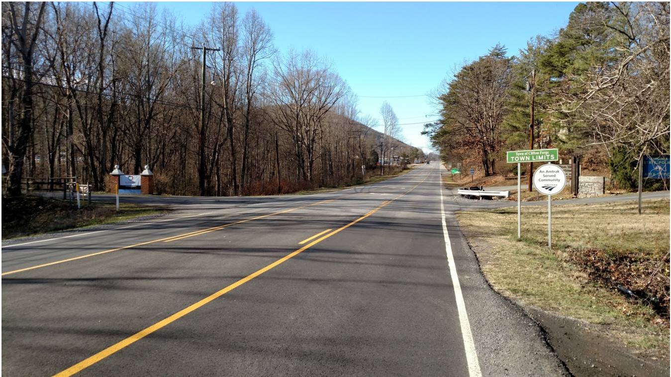
Sidewalk is proposed on the north side (right in photo) of this section of Main St beginning at Oakwood Dr
