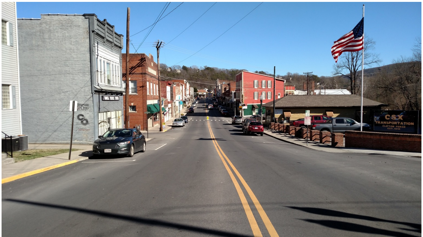
Ridgeway St at Roxbury St facing east – shared lane markings are recommended in both directions
