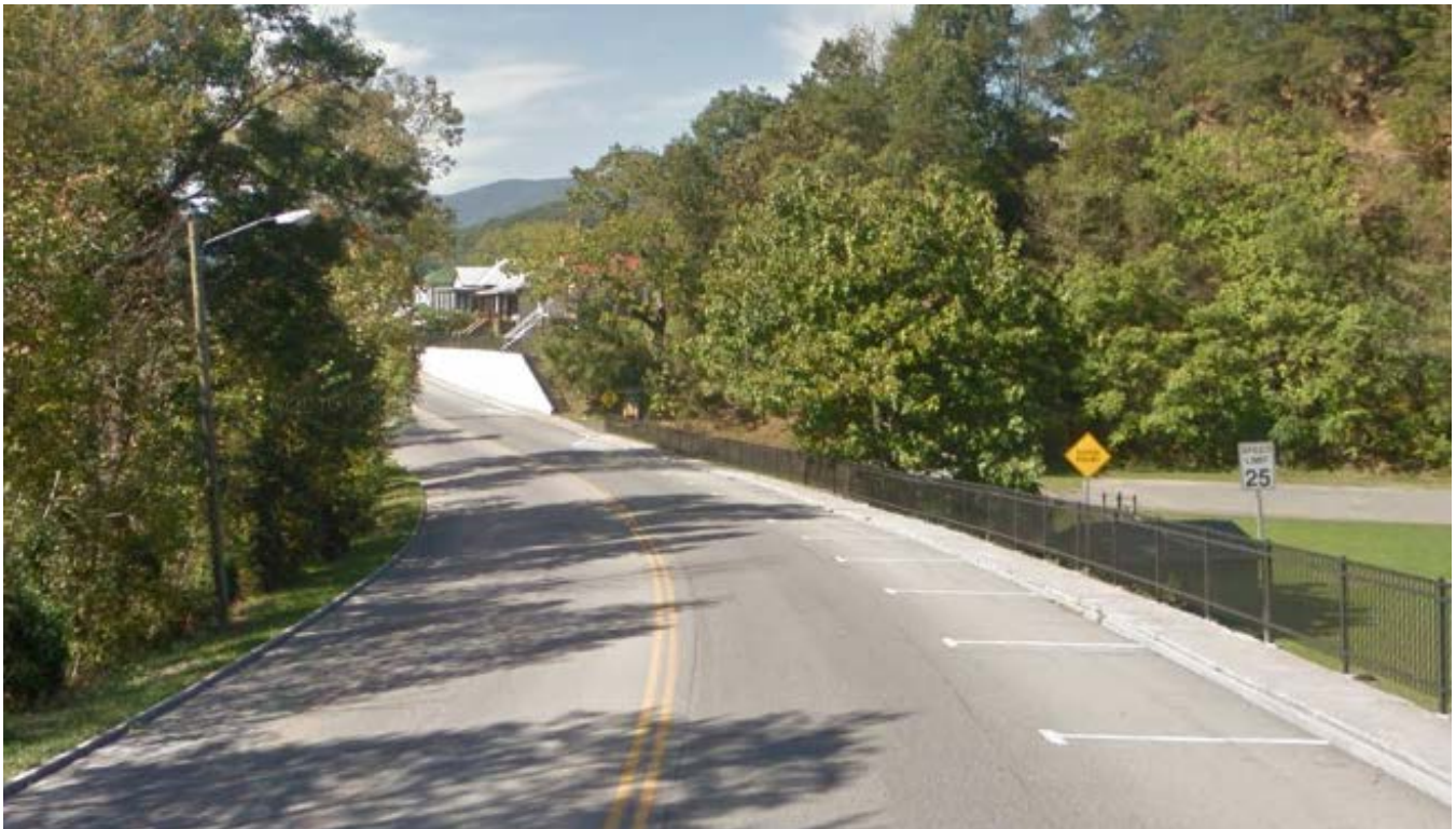
Main St at Booker T. Washington Park facing west – shared lane markings are recommended in the westbound direction (right side in photo) with bike lanes in the eastbound direction (left side in photo) where space allows
