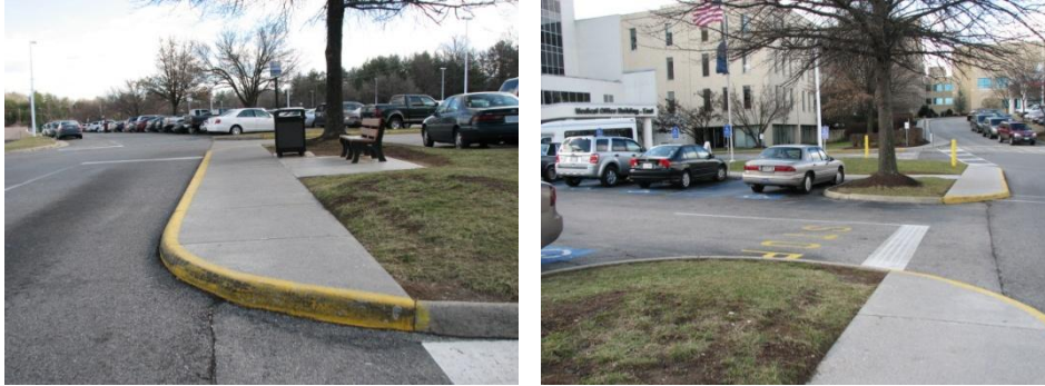
Lewis Gale Medical Center sidewalks around the bus stop need ADA ramps
