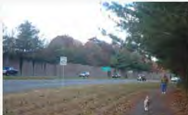
Figure 45 - Fairfax County Parkway. An example of a Multimodal Through Corridor.
