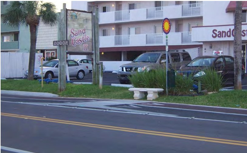
Figure 26: Clear designation for cars, bicyclists (black lane), pedestrians (red lane), and bus riders (bench) with an accessible concrete bus stop landing pad, Reddington Beach, FL
