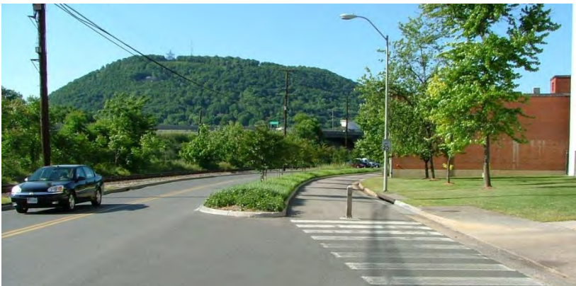
Figure 23: Adding no new impervious surfaces, Williamson Road was redesigned to accommodate pedestrians/bikes within the existing street pavement along a path, the “Mill Mountain Greenway”, separated from traffic by a landscaped median, City of Roanoke
