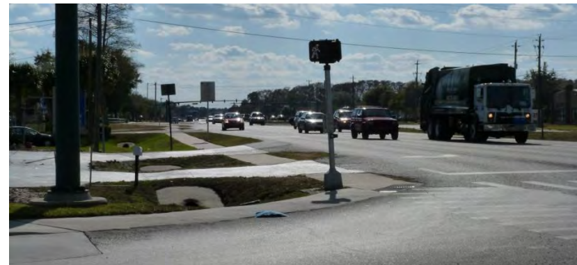
Figure 25: Open drainage channels minimize expenses while still providing space for pedestrians along a 4-lane road, Sanford, FL
