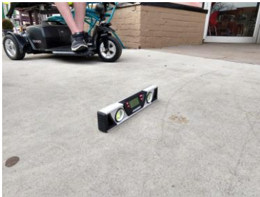
Figure 5. The sidewalk has been ramped up to the entrance, so that the entrance is accessible, but this can result in a steep cross slope difficult to navigate.
