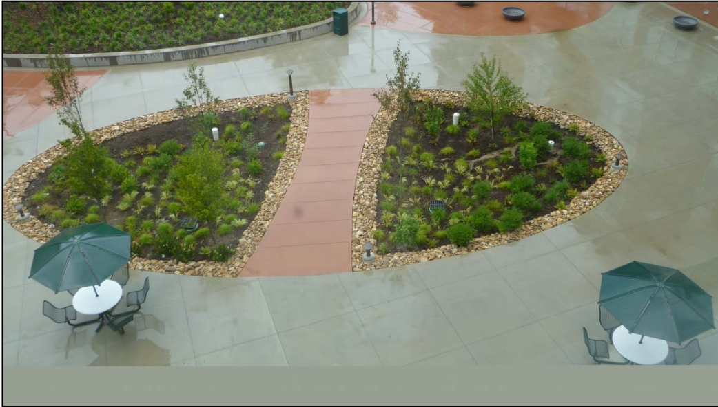
Courtyard Rain garden at Virginia Western Community College (Picture courtesy of City of Roanoke)
