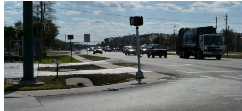
Figure 25: Open drainage channels minimize expenses while still providing space for pedestrians along a 4-lane road, Sanford, FL
