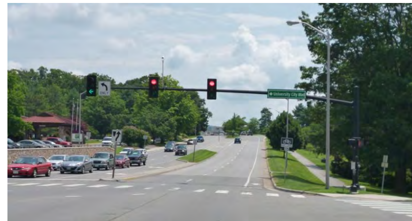
Figure 21: A walking path is separated from the busy 4-lane roadway by a grass buffer with trees, Town of Blacksburg
