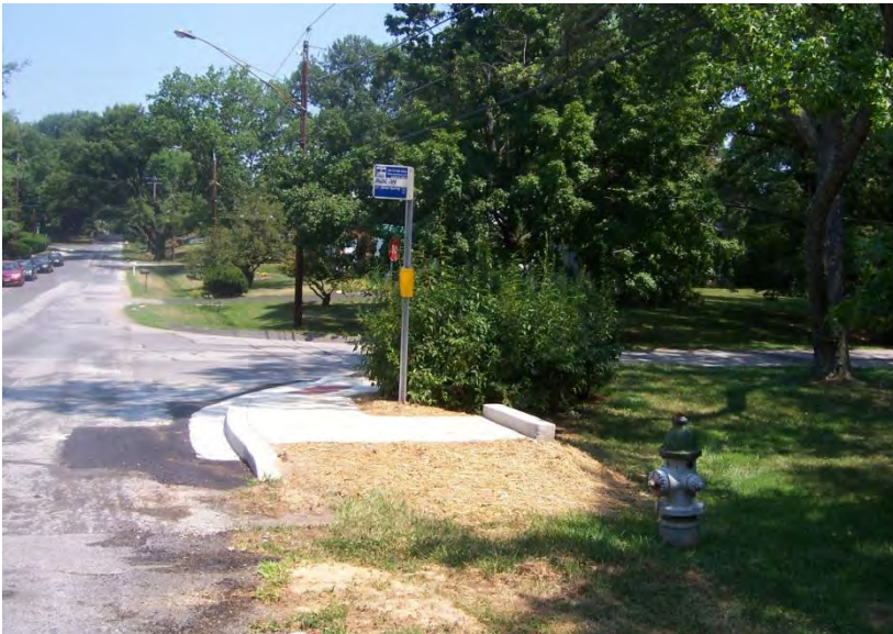
Figure 30: Accessible pedestrian waiting area at a bus stop, Montgomery County, MD
