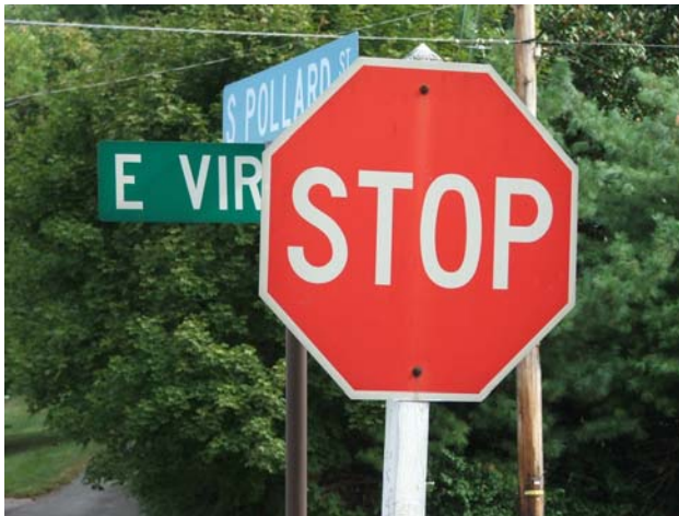
Street sign and stop sign on separate posts. Street sign obscured.
