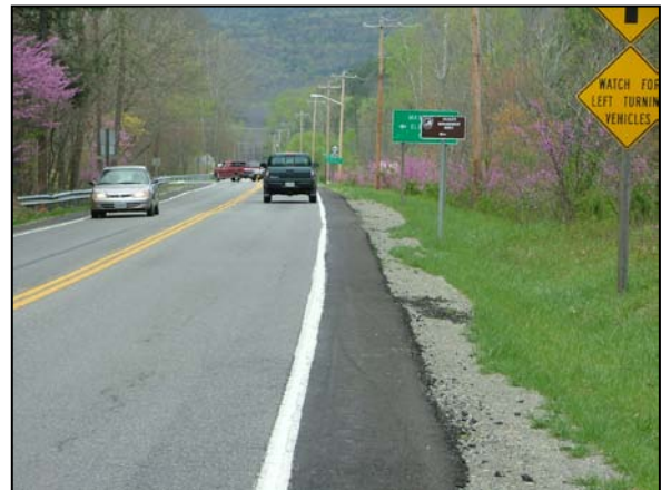
Improved paved shoulder on Route 311 in Roanoke County installed by VDOT in 2011 as part of its maintenance program
