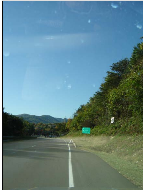
Inconsistent paved shoulder along Electric Road/419 in Roanoke County
