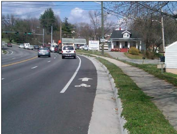
Bicycle lane on Gus Nicks Boulevard (City of Roanoke) installed as part of the 2011 annual paving program
