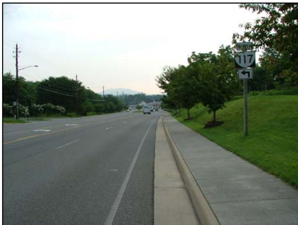
Wider outside travel lane on Brandon Avenue in the City of Roanoke
