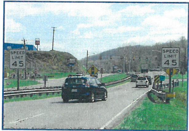
Image 3.1.3 The bridge over Wolf Creek along Washington Avenue is too narrow to accommodate pedestrian or bicycle traffic.
