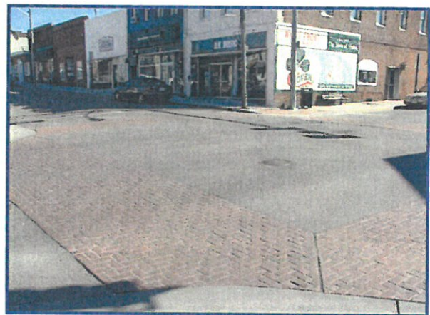
Image 3.3.1 The intersection of Lee and South Pollard Streets is marked with pavers.
